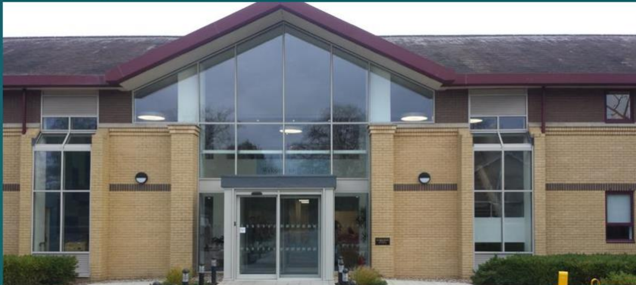
Safety Office at Greenwich House
